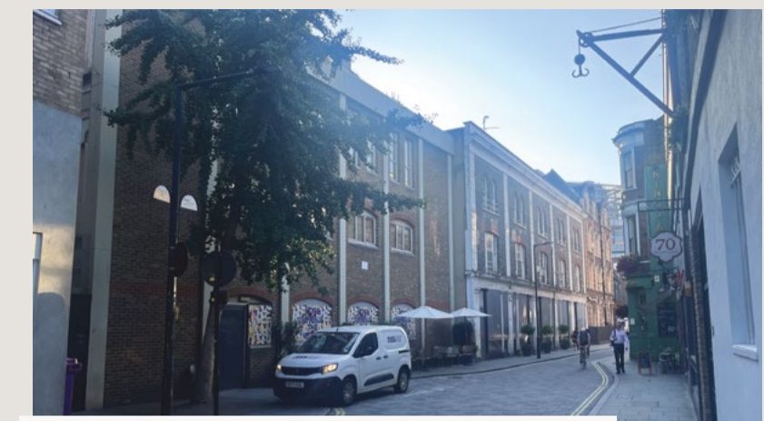
View of 1-9 Newcomen Street from junction with Borough High Street
