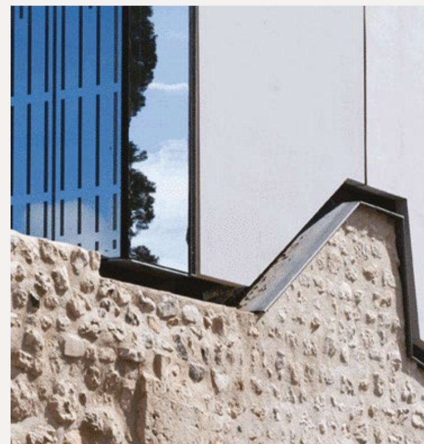
Music School, Louviers (France) by Opus 5 Architects
